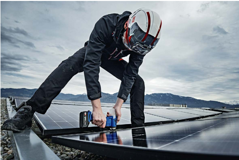
PV module mounting is a vital growth market for riveting solutions.
